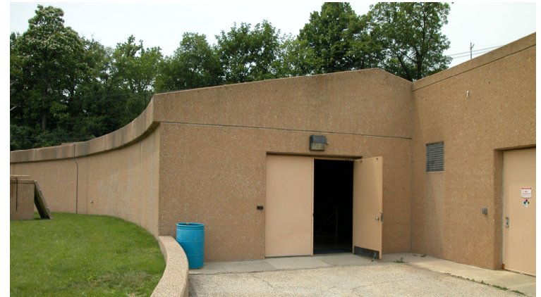
The well house entrance: facing west
