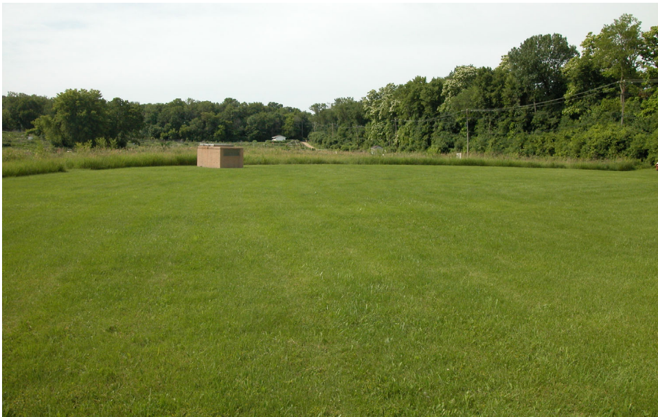
The buried reservoir: facing south
