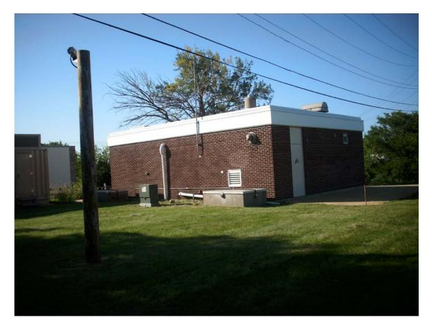
Drilled: 1965 Diameter: 22" Well Depth: 753' Casing Depth: 172' Eau Clarie Depth: 240' (aquitard) Aquifers: Wonewoc and Mt. Simon Formations
