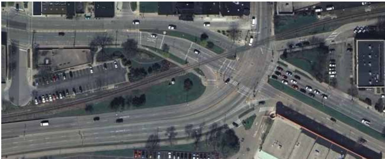
Figure 10. Existing Conditions at the East Gateway
