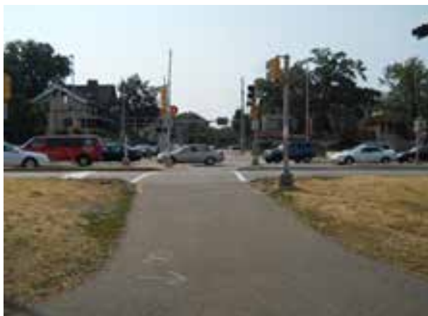
Figure 3. Broom Street and John Nolen Drive Intersection Looking North from Capital City Trail
