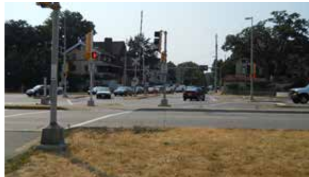
Figure 4. Broom Street and John Nolen Drive Looking North from Law Park
