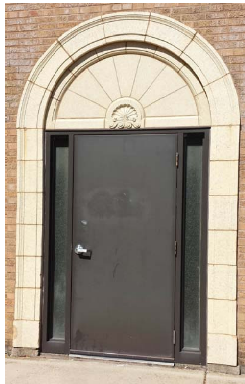
02 EXISTING DOOR to LOWER LEVEL
