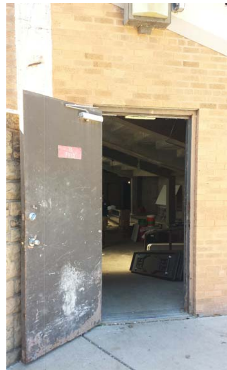
03 EXISTING SERVICE DOOR to LOWER LEVEL
