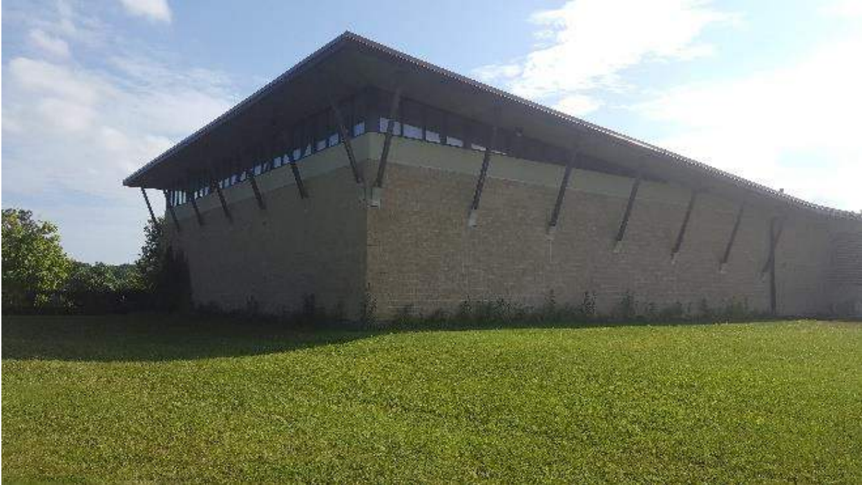
Figure 9: Northeast corner of gymnasium.
