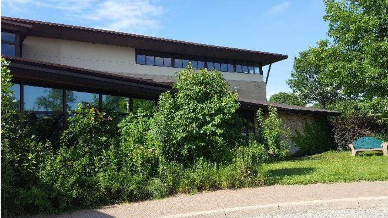
Figure 6: WPCRC southeast corner and south wall of gymnasium.
