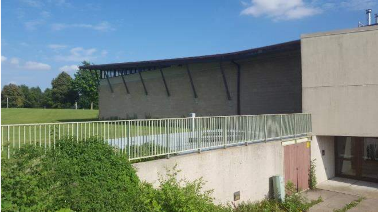
Figure 10: North wall of gymnasium and chiller pit.
