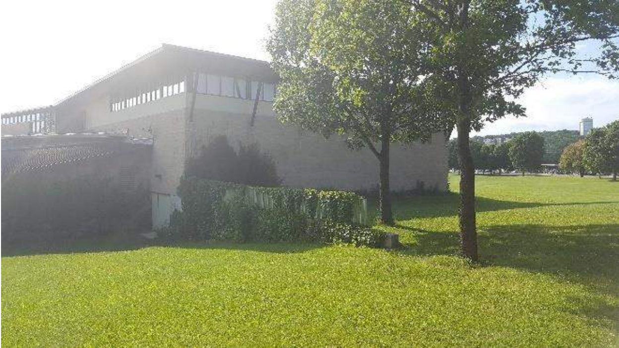
Figure 8: East wall of gymnasium.
