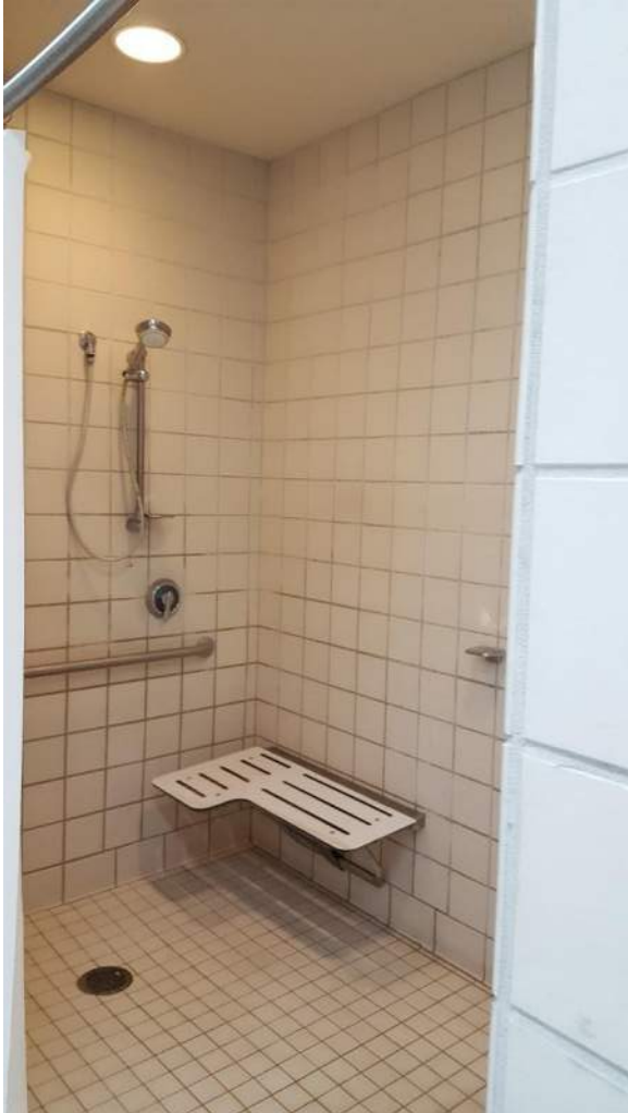
Figure 16: Typical accessible locker room shower stall.
