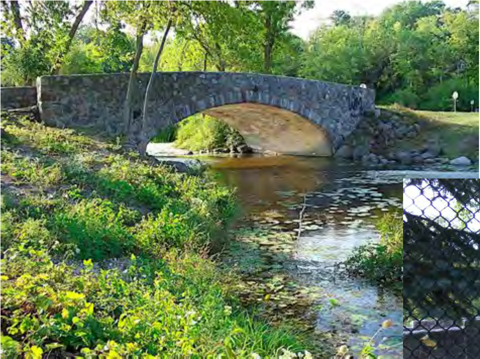
West Bridge along Vilas Park Drive
