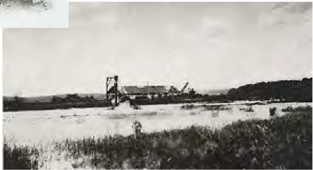
Lagoon Dredging by the La Crosse Dredging Co. 1906
