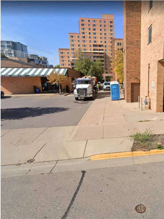
VIEW FROM W. MIFFLIN ST.
