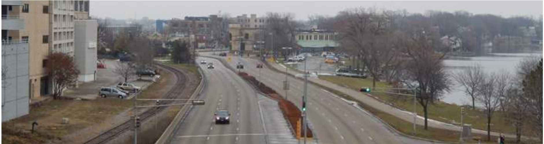
Figure B.35 View Looking East from Monona Terrace Parking Ramp
