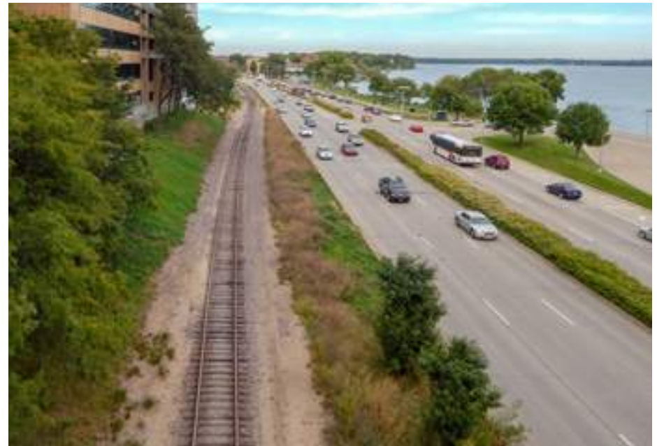
Figure B.24 View from Monona Terrace Parking Ramp Looking East
