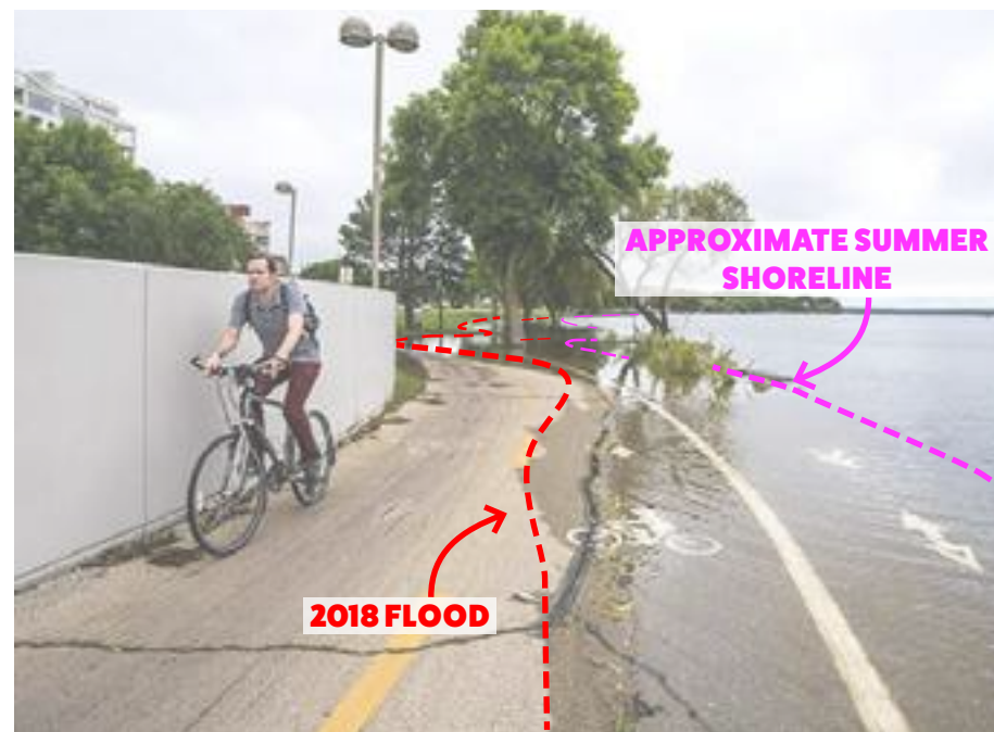
Figure B.42 2018 Flood encroaching on the Capital City Trail
