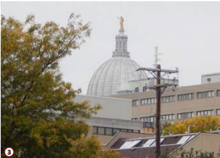
Figure B.9 Blocked Capitol View from Law Park
