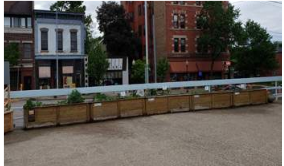
Figure B.17 Community Garden - MWU Water Reservoir Roof at 201 S Hancock St.
