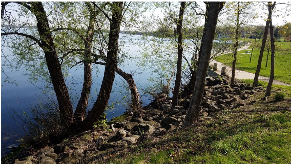
The wetland is located at the water's edge, with rock riprap occurring above the wetland boundary.
