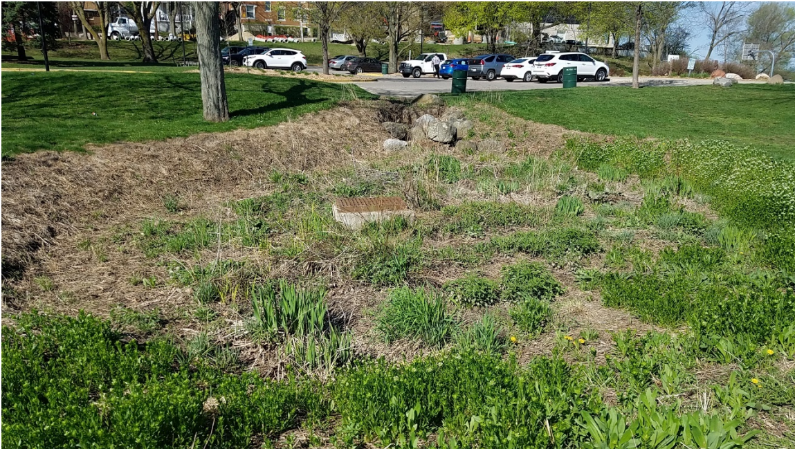
A constructed detention basin contains wetland vegetation.
