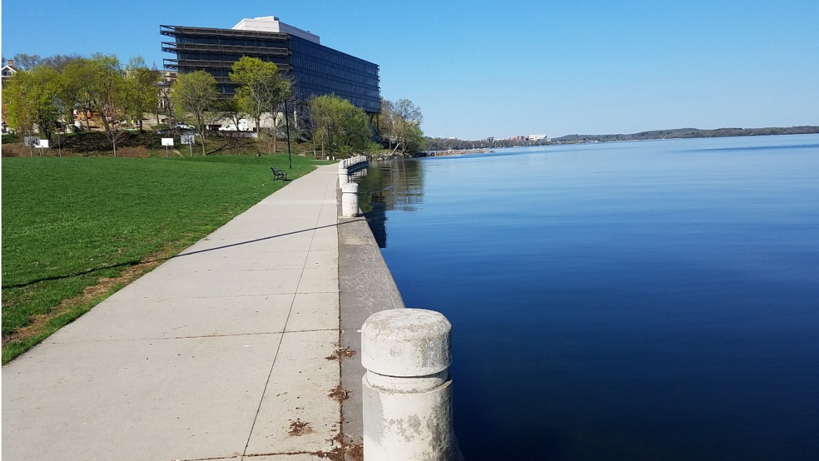
The majority of the shoreline is lined with a concrete wall.
