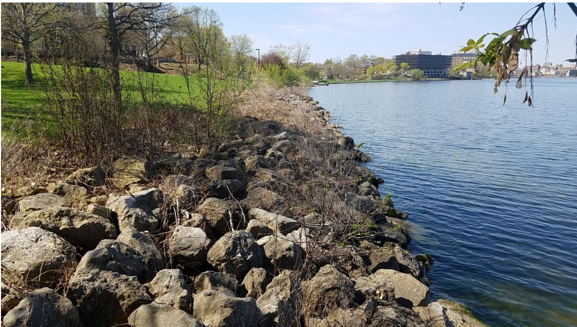
The northeastern half of the shoreline is lined with large boulders on a steep slope.
