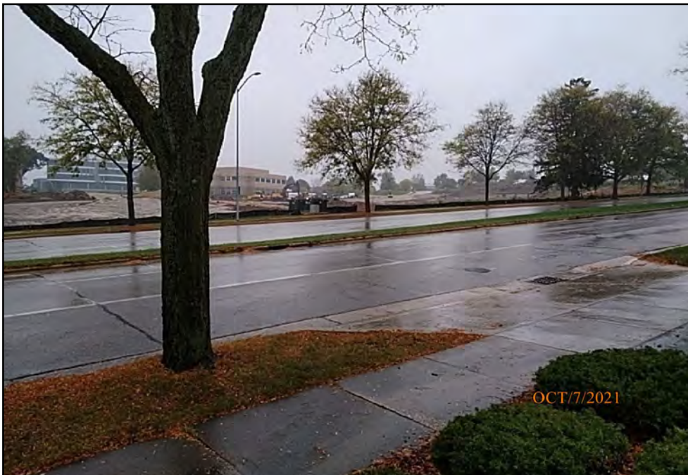
Appendix A-11. Site 47DA0817 Construction South of Mineral Point Rd. at East Edge of Site, View Southwest
