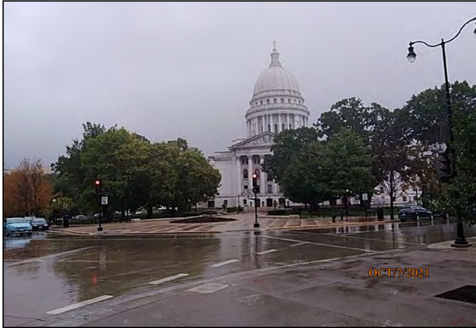
Appendix A-18. Site 47DA0868 (Capitol Building) from Intersection of W. Main St. and S. Carroll St., View North
