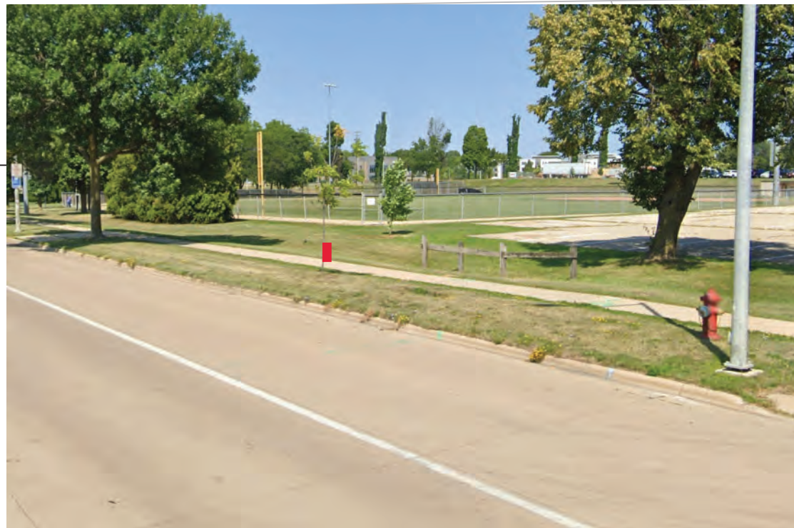
Small Tree Removed
