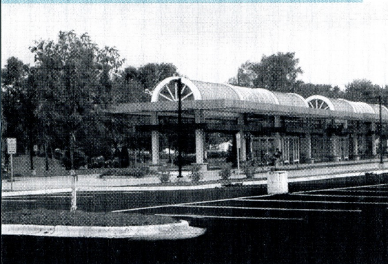
New North Transfer Point Park & Ride Lot
