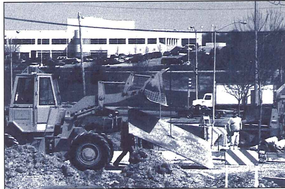
Construction begins on the West Transfer Point.
