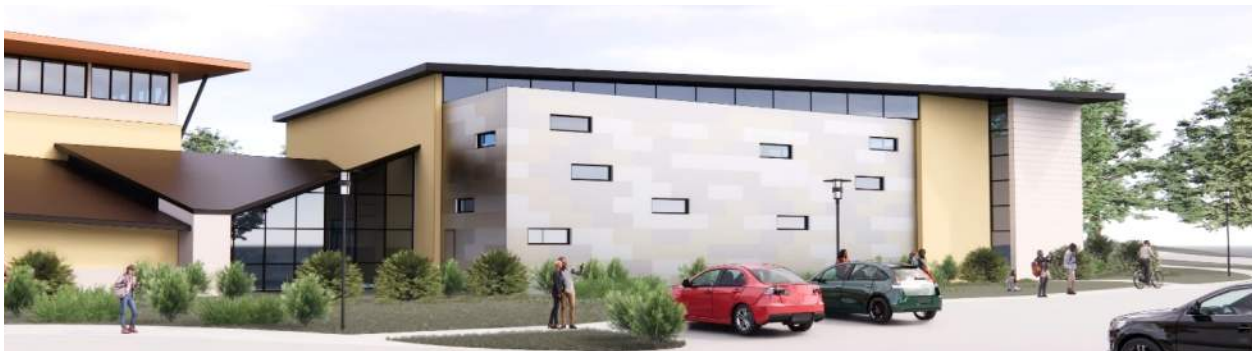
View of Expansion from Southeast
