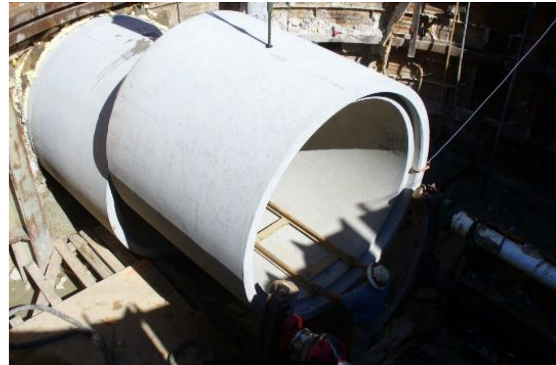
96" pipe tunneling on University Ave, Madison, WI (2013)
