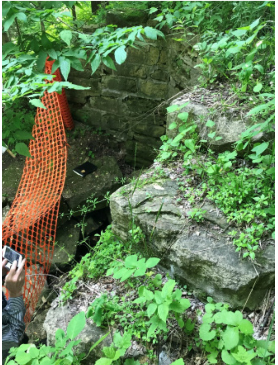
Figure 2: View of capstones and minimal overburden above the wing walls (additional soil over the ventral arch wall.)
