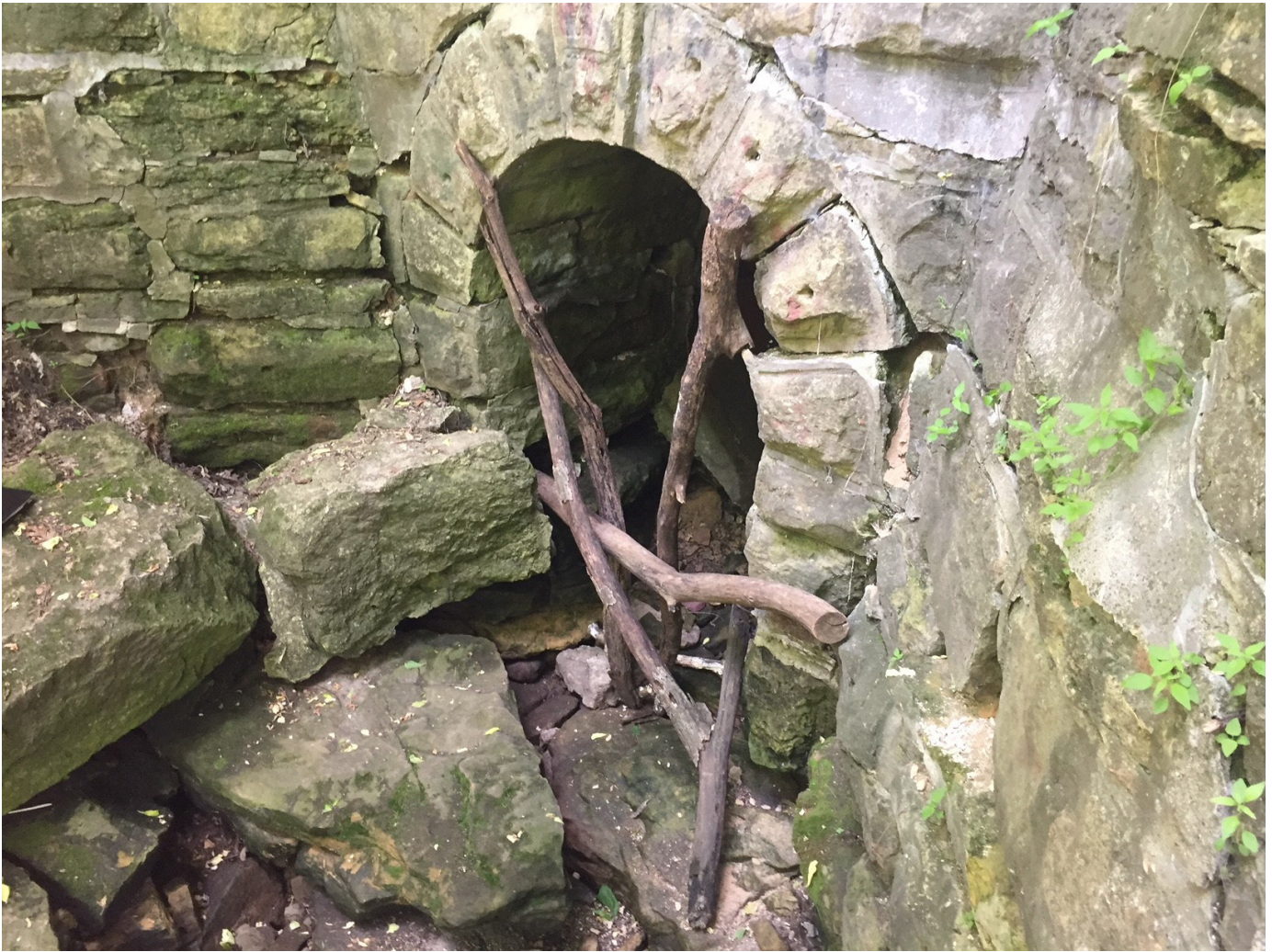
Figure 3: Overall view of arch.
