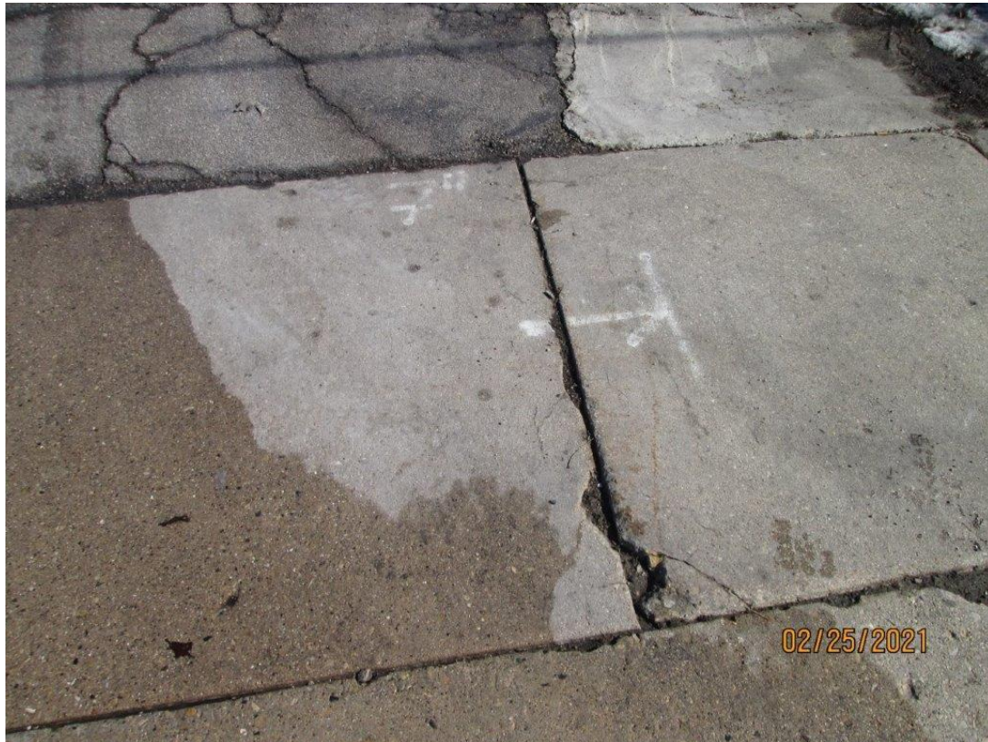
Voids and Erosion of Joints
