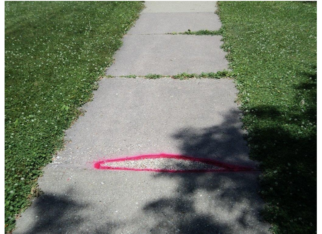
Voids and Erosion of Joints
