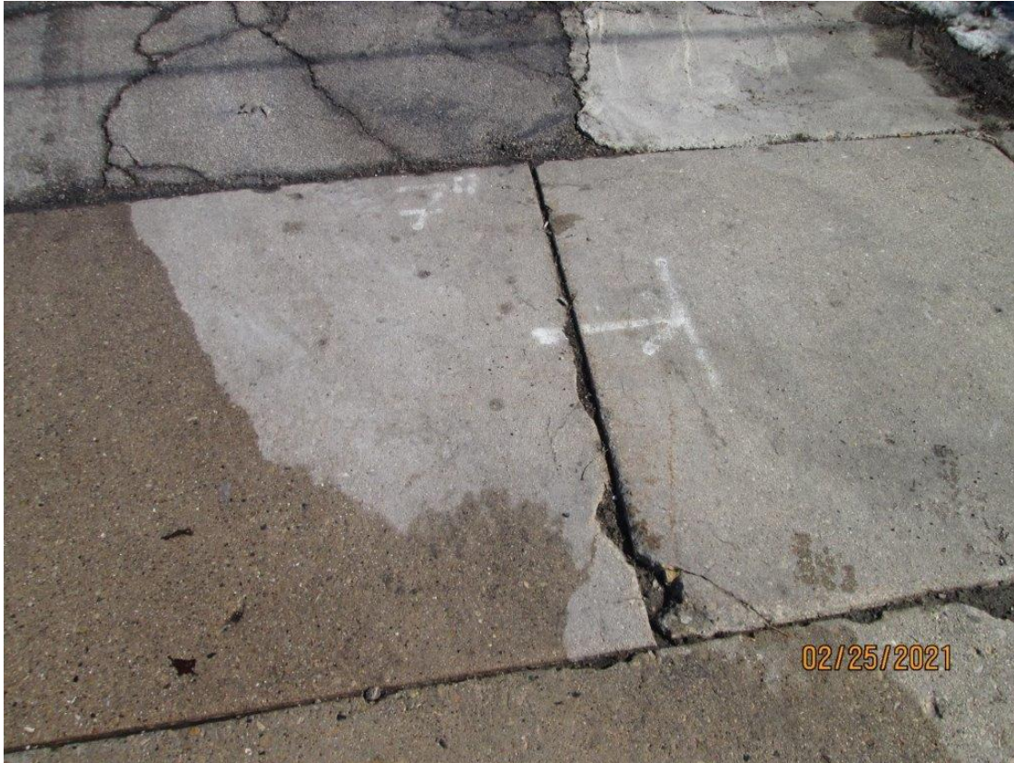
Voids and Erosion of Joints
