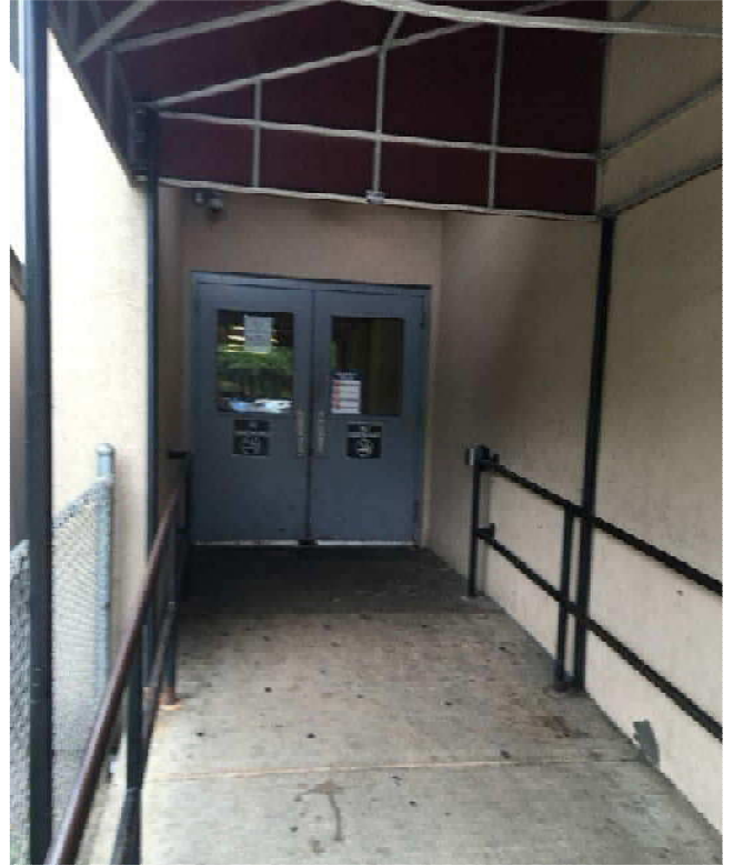
Entrance to shelter
