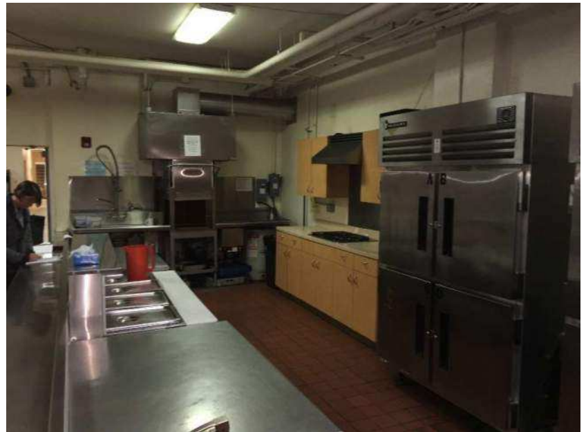
Kitchen – dishwashing area and warming stove
