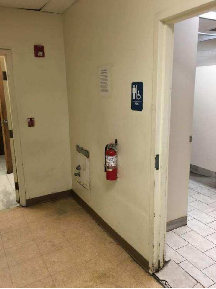
Entry to main restroom
