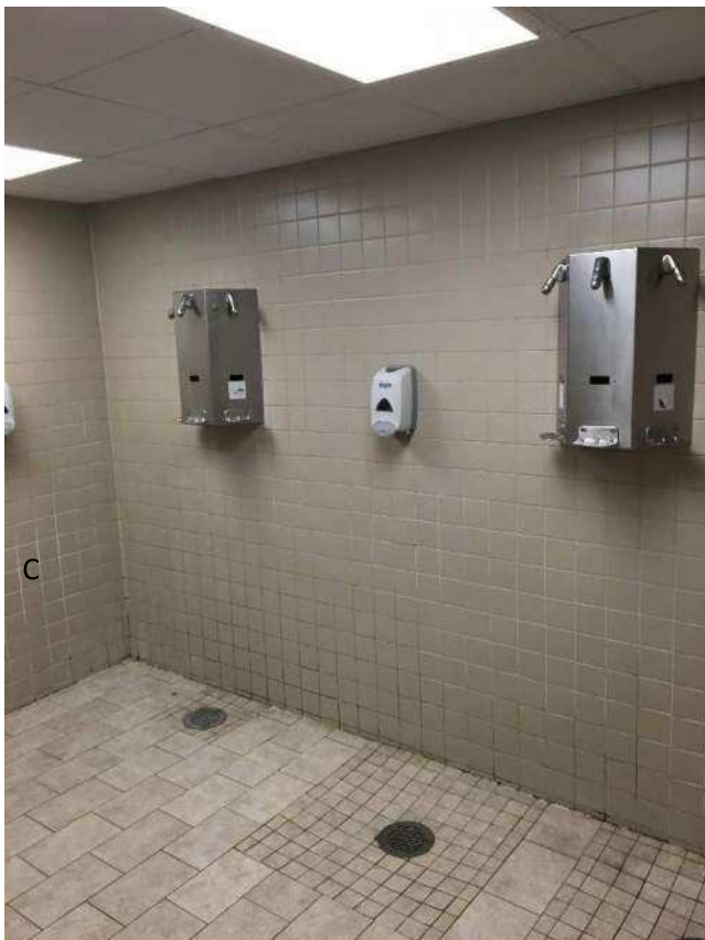
Showers in main restroom area
