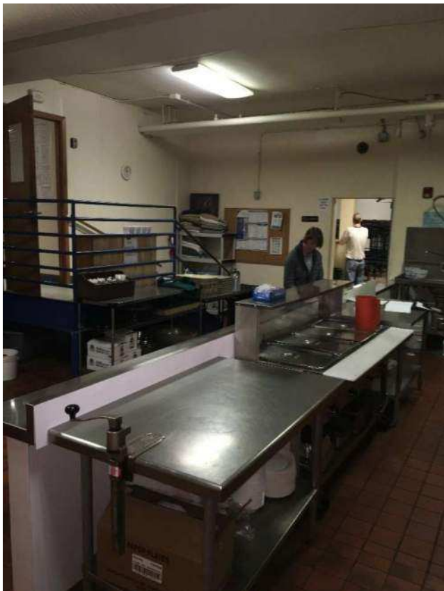
Serving line in Kitchen – stair to office beyond
