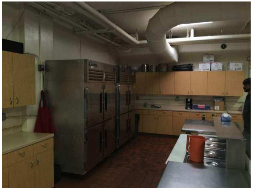
Kitchen – refrigerators and storage areas
