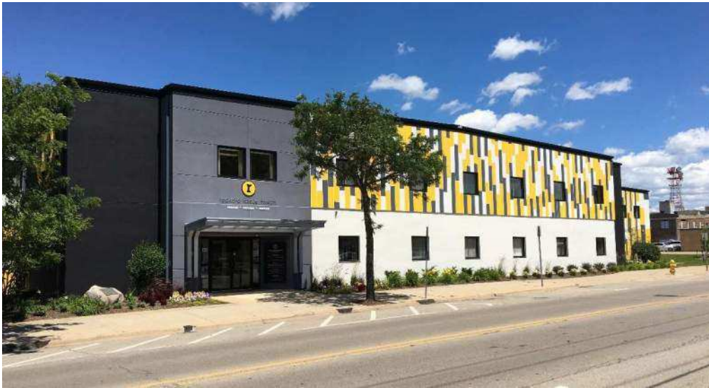
Main entrance to building reception and staff offices
