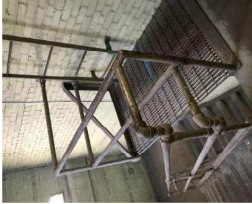
Figure 47 – Roof hatch access
