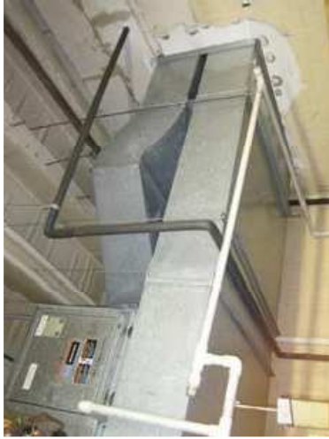
Figure 129 -- AHU-1 Ductwork
