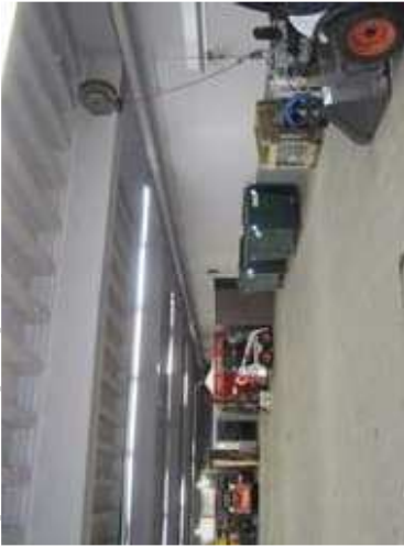
Figure 264 Lighting with Occupancy Sensor
