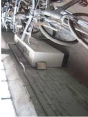
Figure 120 – Convector Unit
