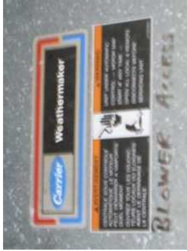
Figure 143 – Make-up Air Unit Nameplate
