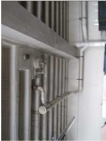
Figure 437 - Sanitary to Floor Drain Above
