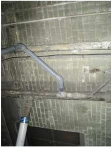
Figure 456 - New Extended Water Service
