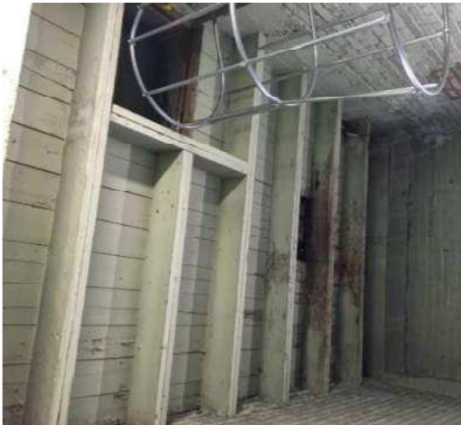
Figure 16 – SW Stair Roof
