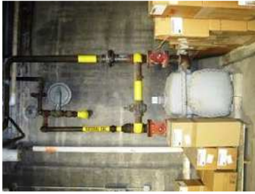
Figure 464 - Gas Meter
