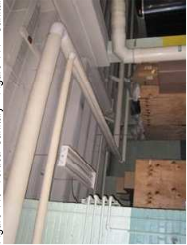
Figure 443 - Vertical Sanitary
