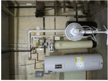
Figure 408 - Water Heater
