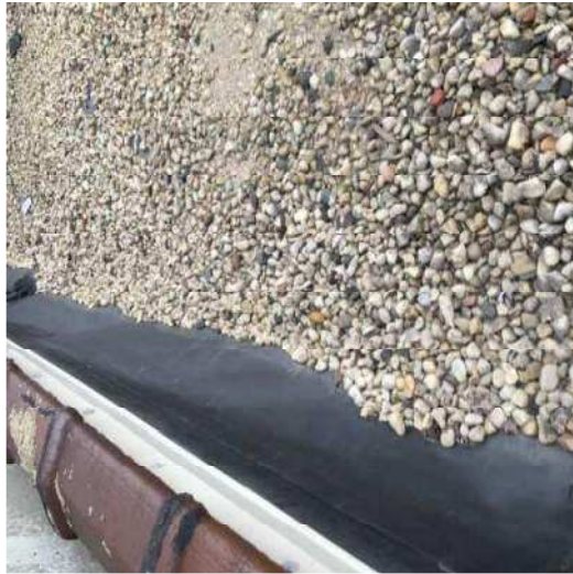
Figure 41 – Roof edge @ parking garage
