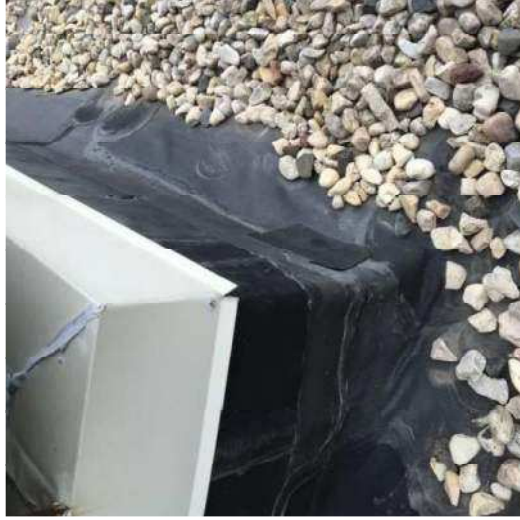
Figure 42 – Flashing curb detail
