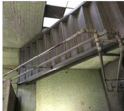
Figure 19 – SW Stair Railing
