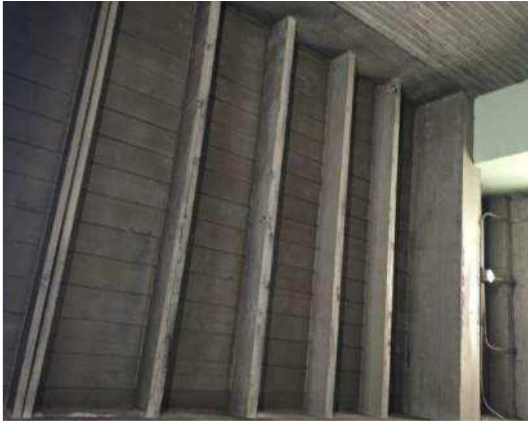
Figure 17 – NE Stair Roof
