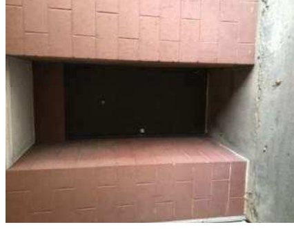
Figure 15c – Ground floor entry door
