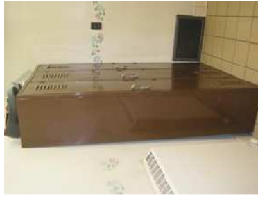
Figure 121 – Convector Unit
