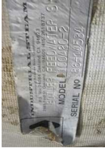
Figure 108 – Feedtank Nameplate
