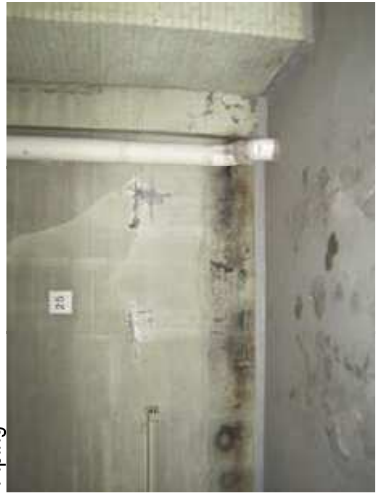
Figure 444 - Storm Piping to Below Grade
