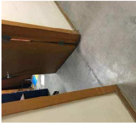
Figure 63 – Conc floor cracks
