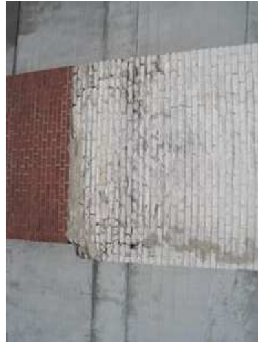
Figure 188 – Masonry Chimney for Boilers
