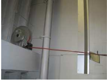
Figure 429 - Compressed Air Reel
