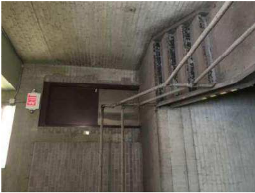
Figure 22 – NE Stair Railing at landing
