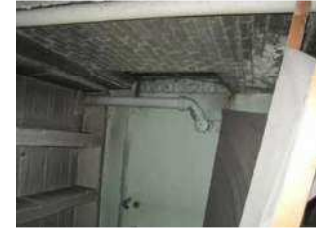
Figure 453 - Storm Discharge
