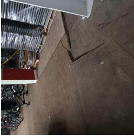
Figure 70 – Concrete slab offset with ramp
