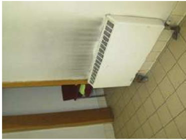
Figure 115 – Convector Unit
