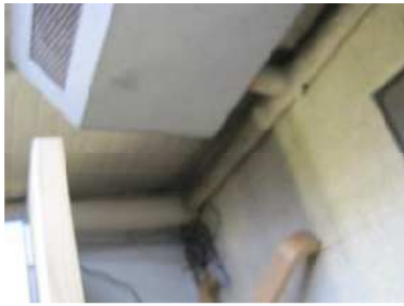
Figure 117 – Convector Unit
