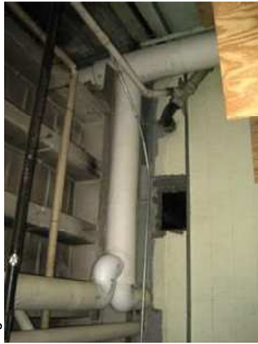
Figure 459 - Horizontal Sanitary Piping
