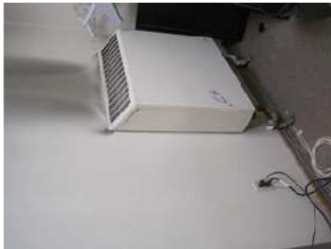
Figure 113— Convector Unit
