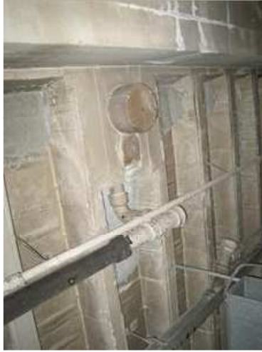
Figure 450 - Sanitary Piping Serving Above
