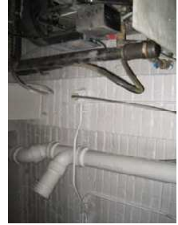
Figure 425 - Storm Piping
