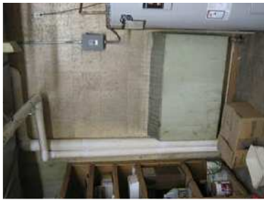
Figure 114 – Convector Unit
