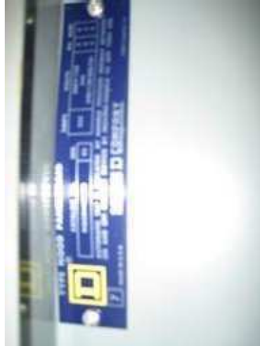
Figure 245 Panelboard Identification
