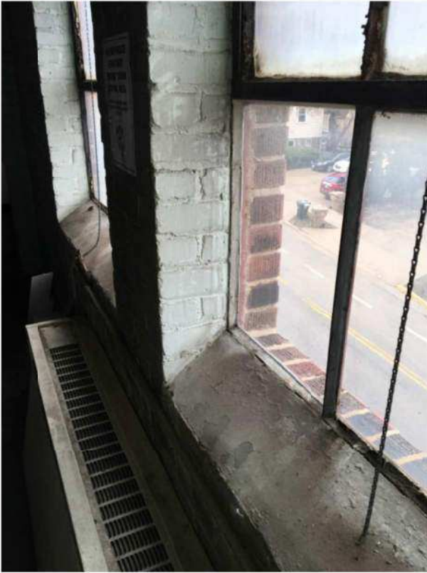
Figure 6 – Exterior window & wall thickness detail
