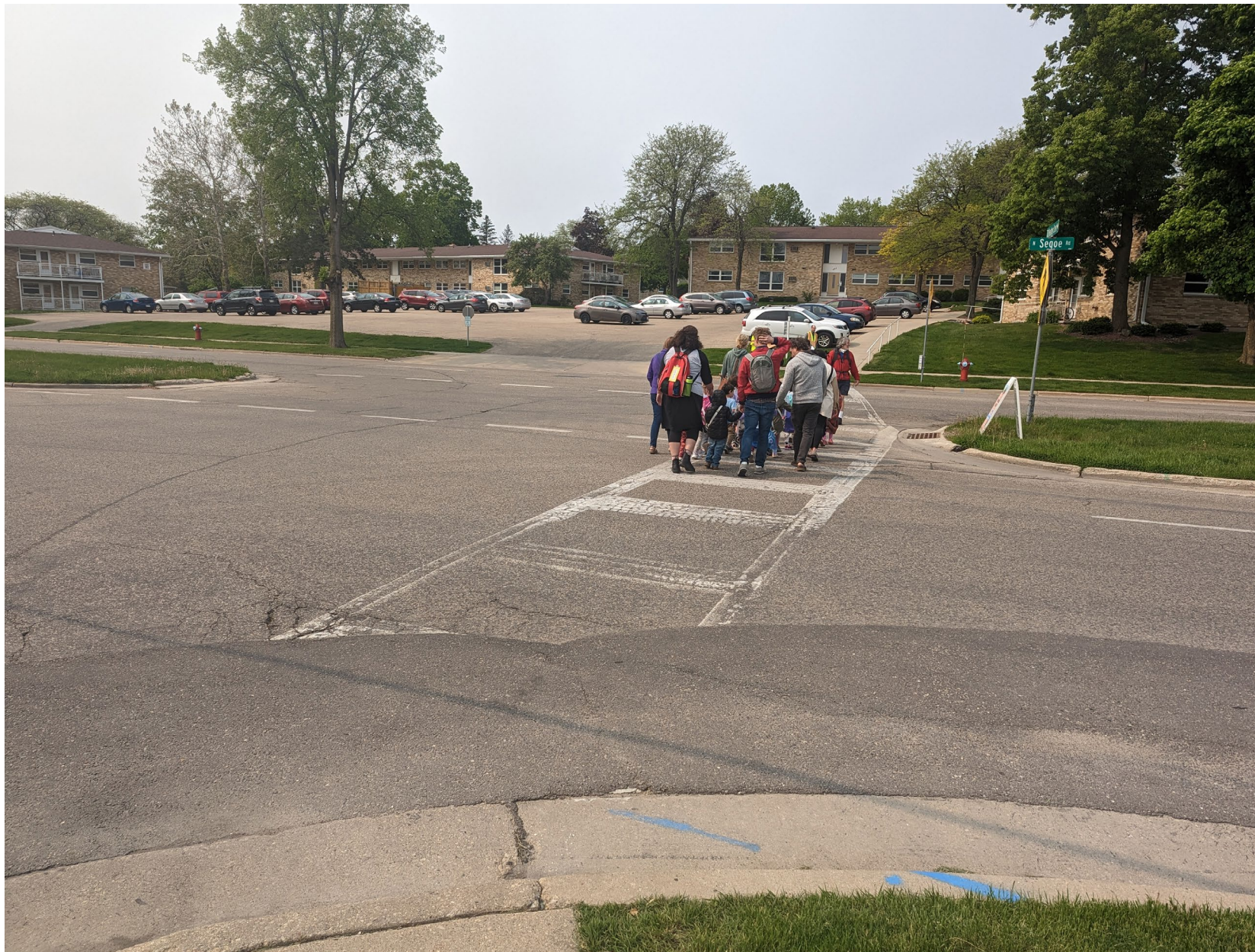
Unsafe Crossing on Segoe Rd: Adults needed to stand in the road and stop traffic to allow children to cross
