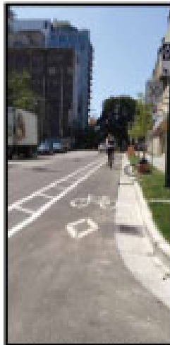
PAINT BUFFERED BIKE LANE
