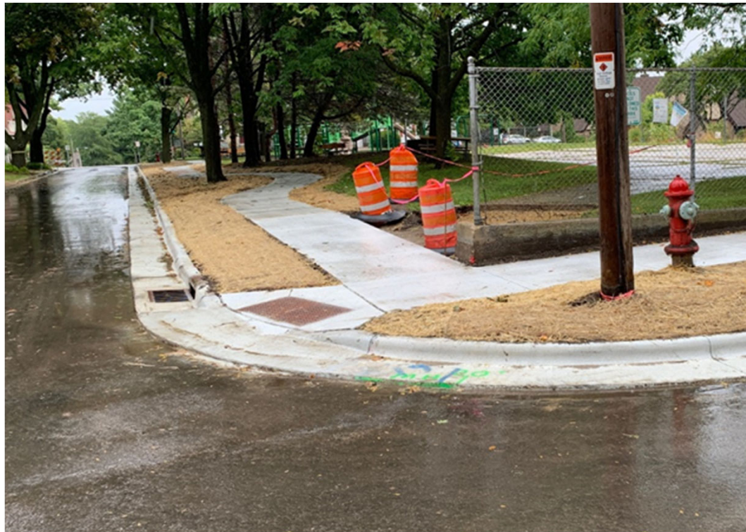
CROSS AND WESTERN INTERSECTION AFTER STREET RECONSTRUCTION
