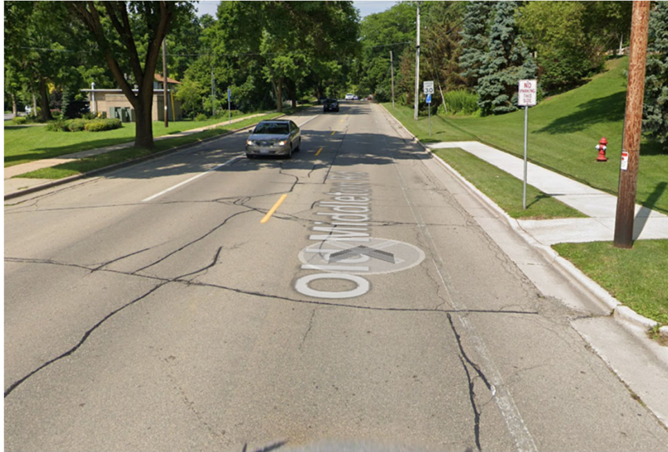
Old Middleton/ Gettle intersection - Northbound
