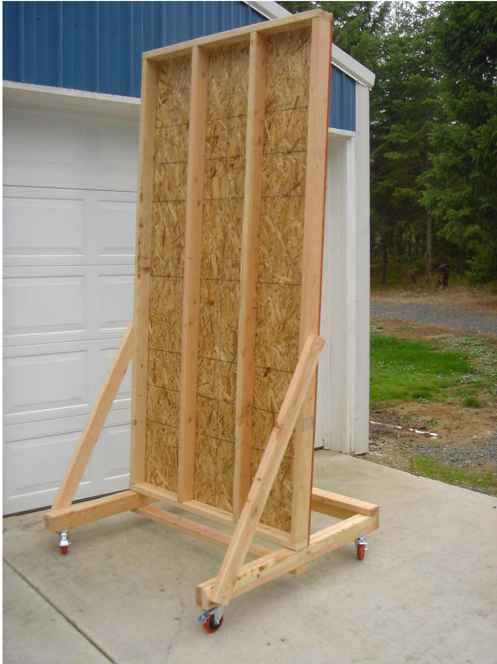
Figure F-1 Simulated wall section prior to installation of insulation, sheetrock and stucco lath (netting).
