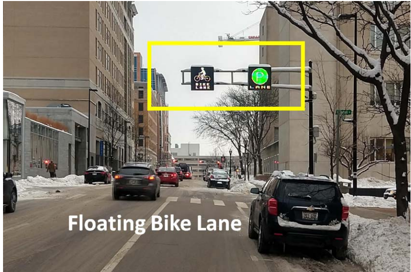
Figure 2.3-2 Floating bike lane on Doty Street. Location of bike lane varies with parking restrictions.
