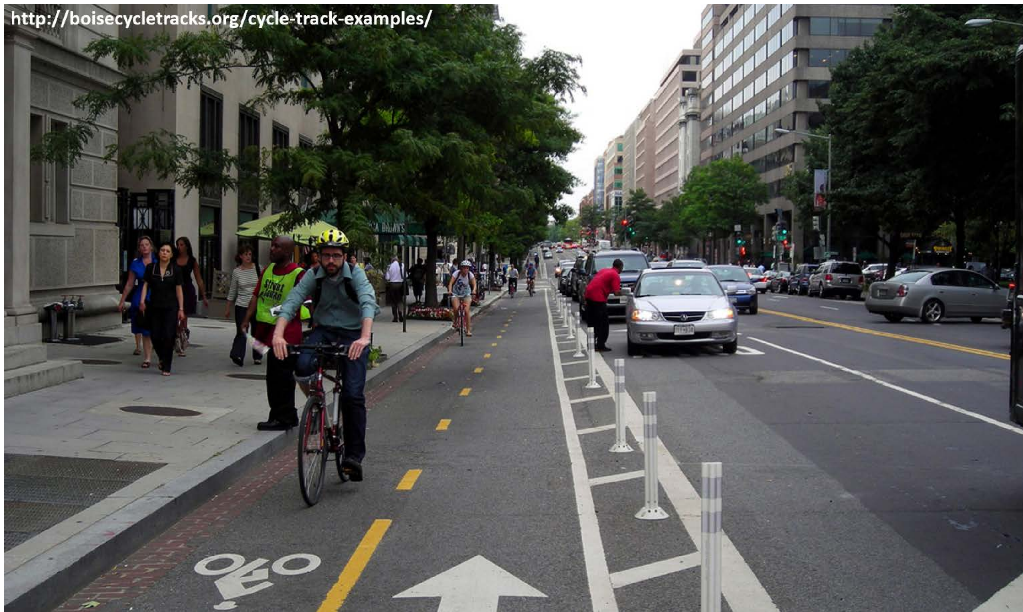
Example of a protected bike cycle track with buffer and flexible delineators in Boise, ID
