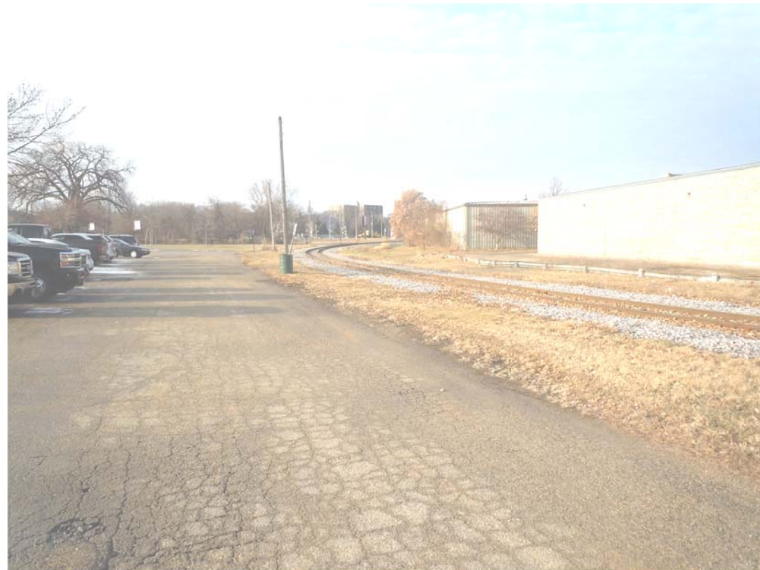
EXISTING PARKING LOT FACING NORTH
