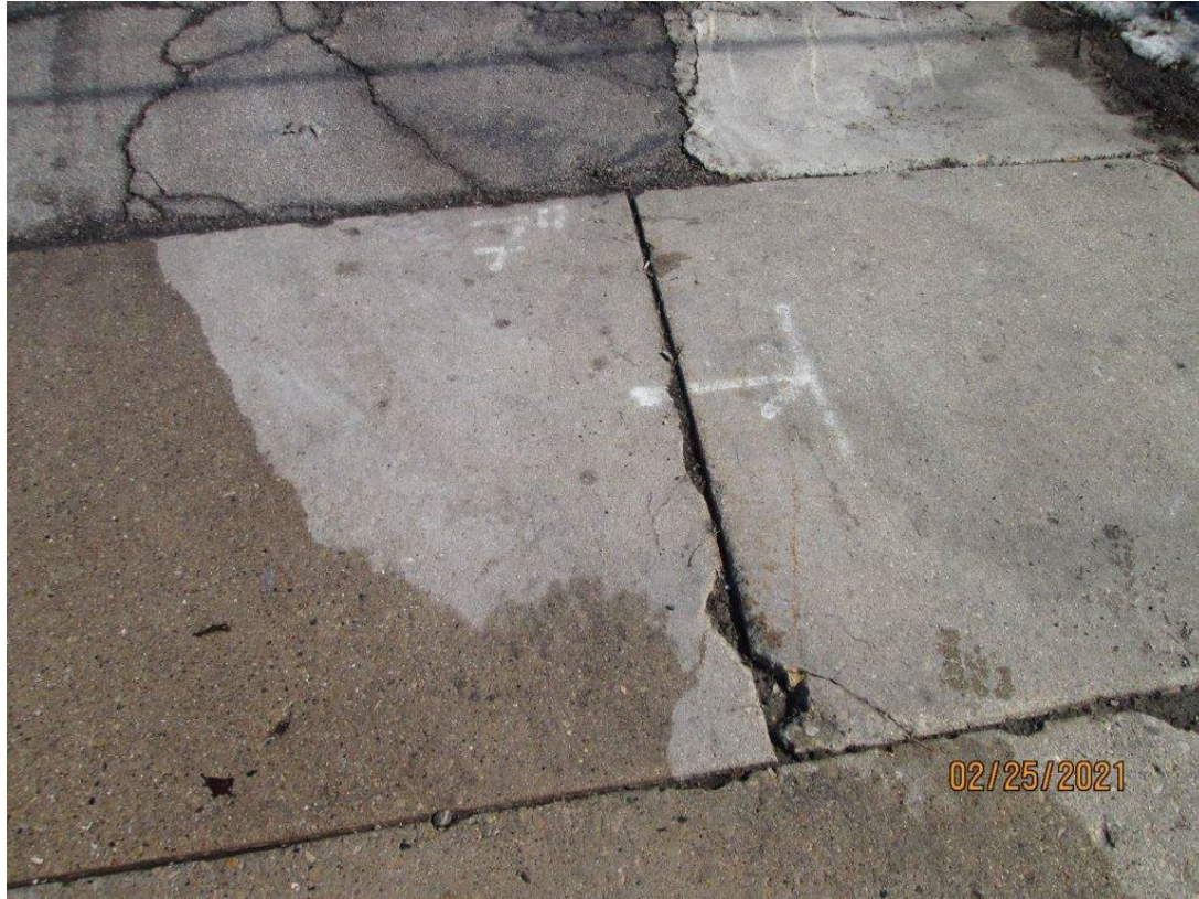
Voids and Erosion of Joints
