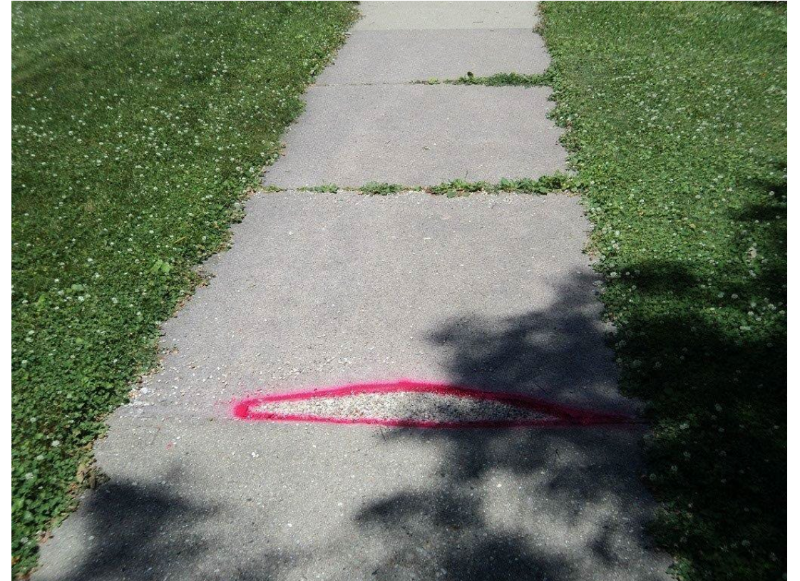
Voids and Erosion of Joints
