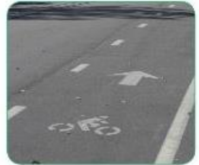
Advisory bike lanes look like dedicated bike lanes, except a dashed line is used in place of a solid bike lane stripe.
