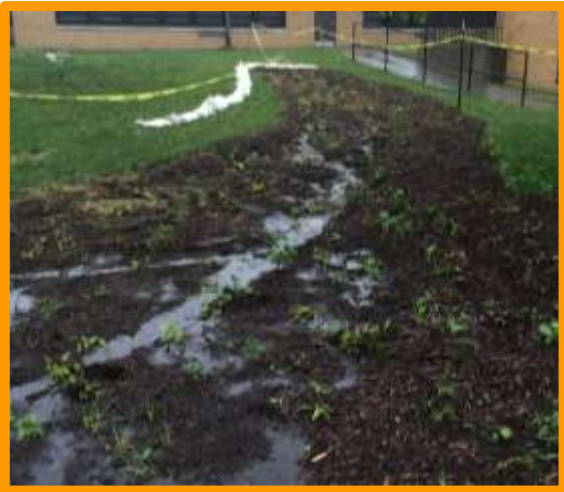
Too much water early on can cause gullying and wash out young plants
